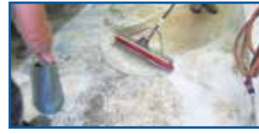
Concrete Clean & Etch
