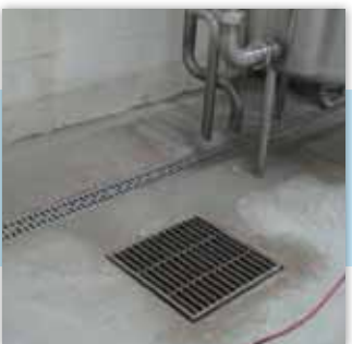
NEW TANK ROOM FLOOR
