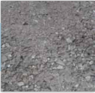
ROUGH CONCRETE SURFACE
