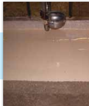
ARMOR-ROCK THX™ Over Old Tiled Manger
