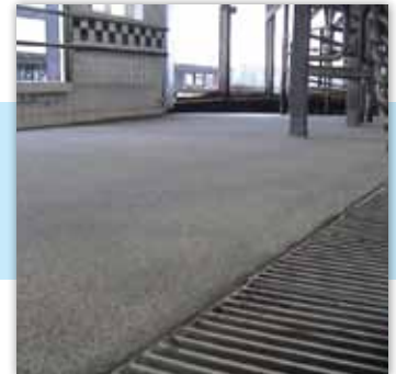
ARMOR-ROCK™ G-DIAMOND Protects New Floor
