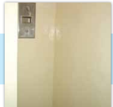
ARMOR-GLAZE™ Restores Wall
