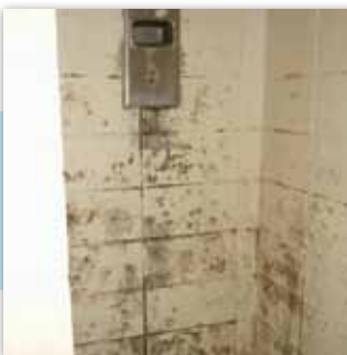
OLD PAINTED BLOCK WALL
