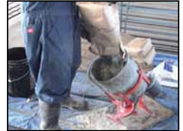
Mix liquids & aggregate
